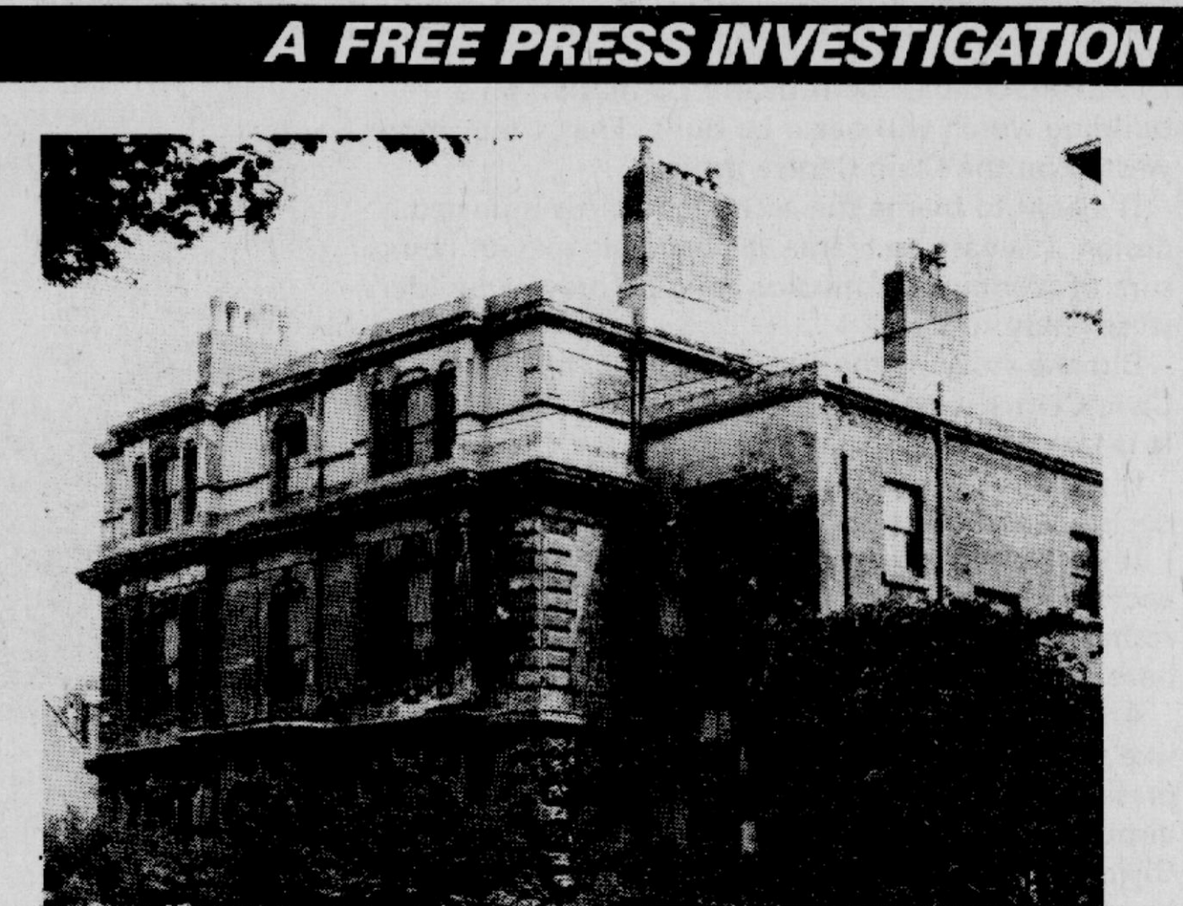
● No. 3 Devonshire Road, Toxteth - the subject of two Notices of Disrepair.
