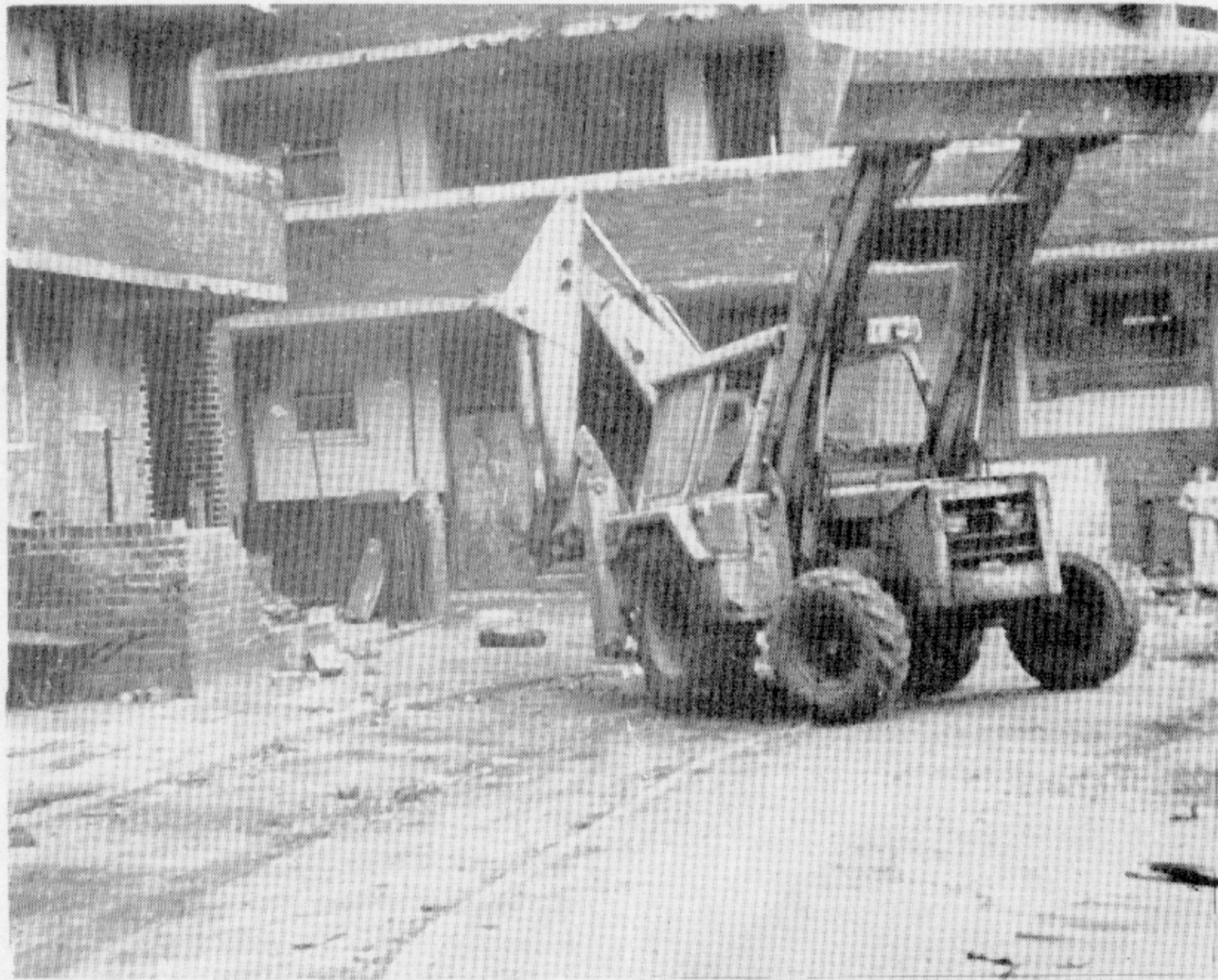
'Improvements' in progress. The flat where the family were barricaded in is on the right.
