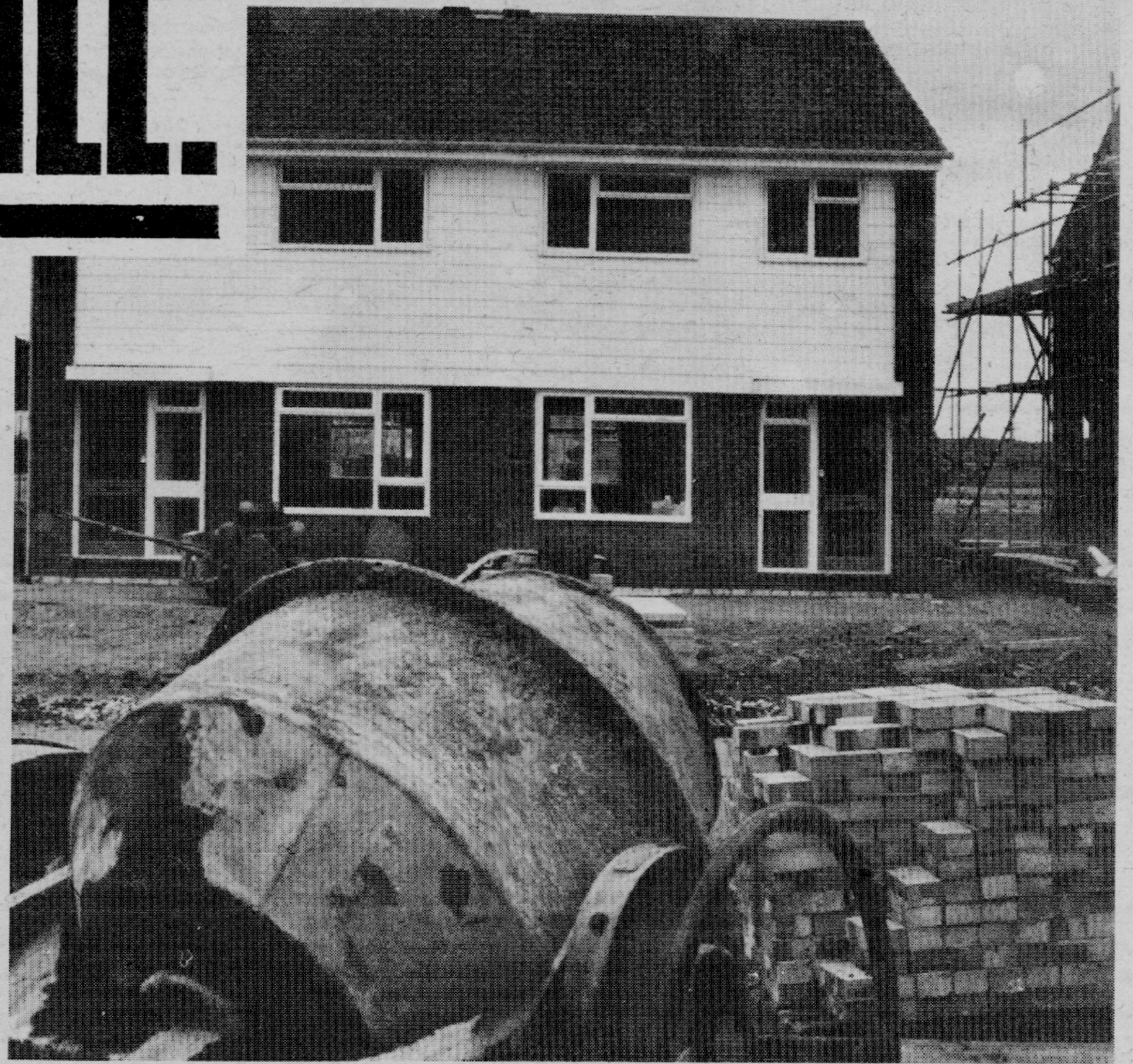
The Stanfield Road site.
